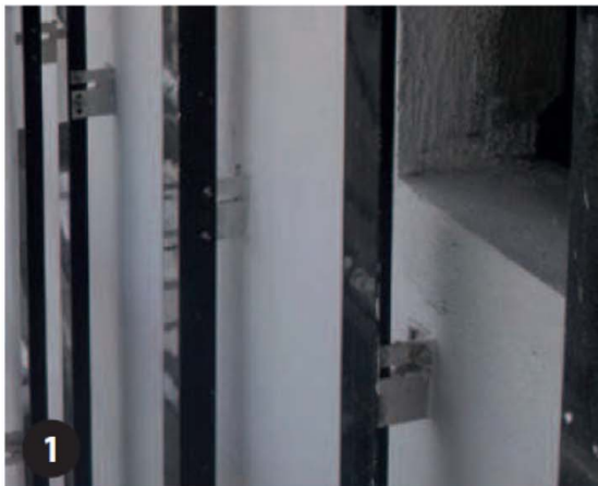
1 butech aluminum profile (L-and T-profile) as facade substructure
