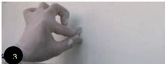
3 Ensure that the facade panel caps are clean and dry before fixing.
